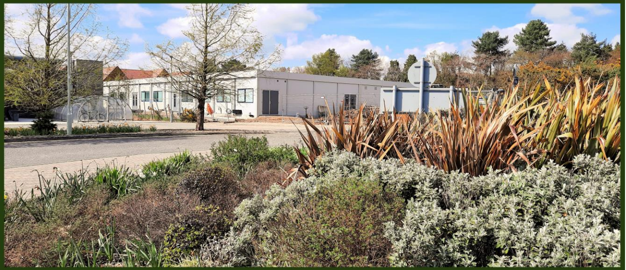
Renal Unit construction viewed across main island
